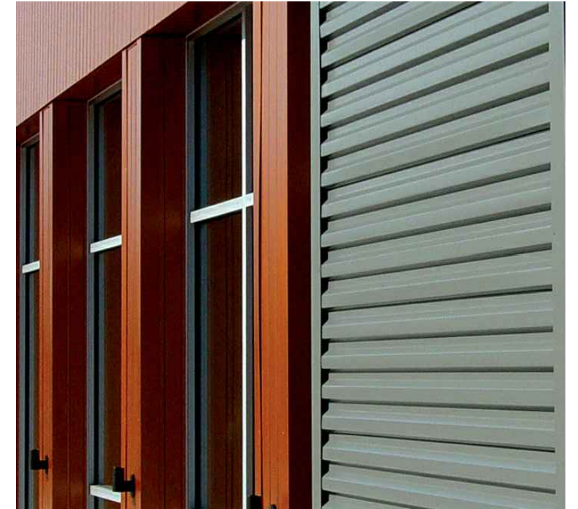
Corrugated Metal Panels installation example
